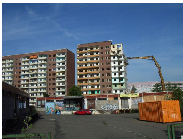
Fig. 7. Demolition of a large block, 2008. Photo: Kabisch.
